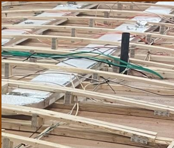
16" On Center Trusses
